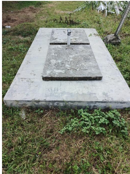
Figure 5. Inspection of Liquid Waste and B3 Waste Management System
