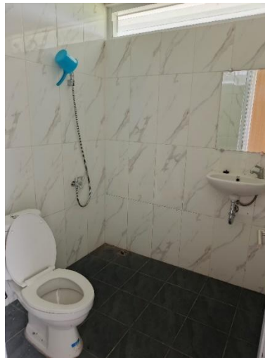
Figure 4. Plumbing and Sanitation System Inspection
