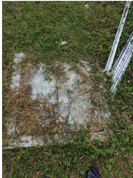
Figure 7. Drainage System Inspection
