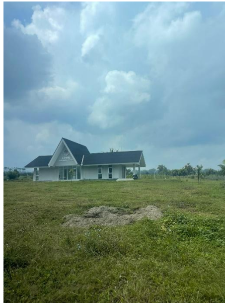
Figure 8. Green Building System Inspection
