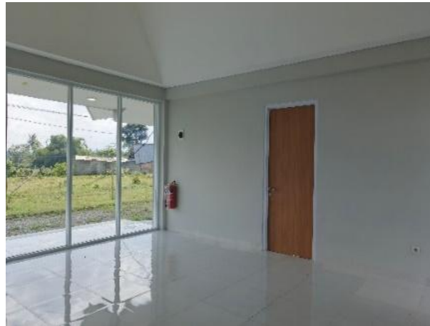
Figure 6. Building Material System Inspection
