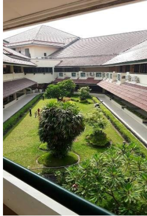
Gambar 15: Panoramic View from 2nd Floor Balcony (Source: Researcher Documentation, 2025)
